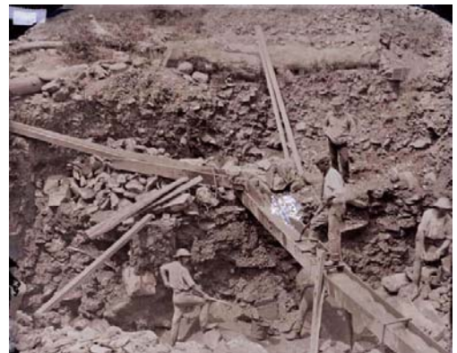
Gold miners working box sluice at end of a wooden race Victoria, circa 1861
