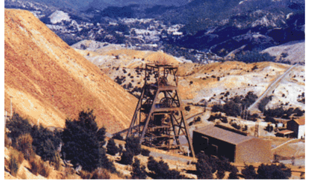
Mt Lyall mine, Queenstown, Tasmania.
