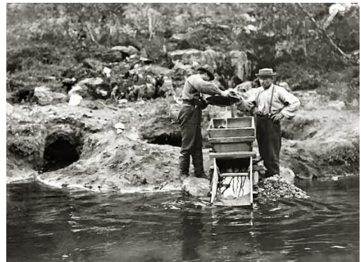
Placer gold winning at Ivalojoiki, near Kultala, in 1898. Photo: Emil Sarlin, GTK.
