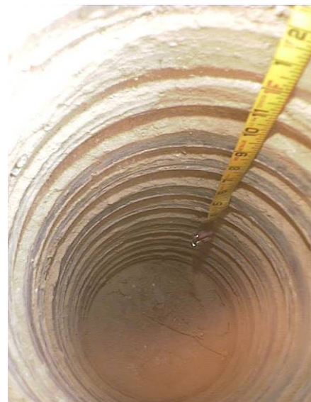
Diamond drill borehole
