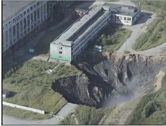
View of the sinkhole at the Berezniki Potash Mine. The collapse was caused by flooding of the underground mine.
