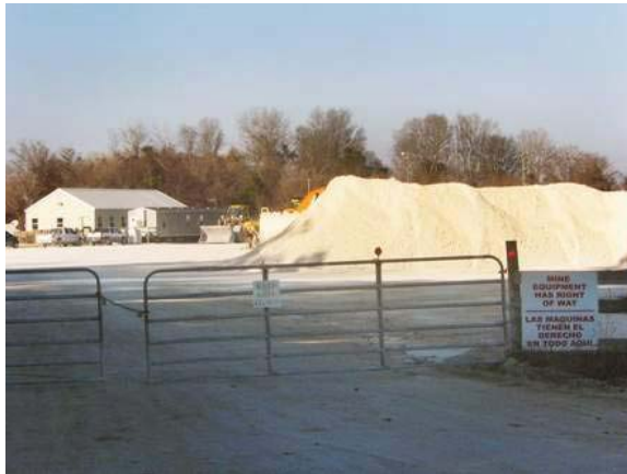
The entrance to the Mazak Mines site in Webster is shown in this Dec. 23, 2010 file photo. (Austin L. Miller)
