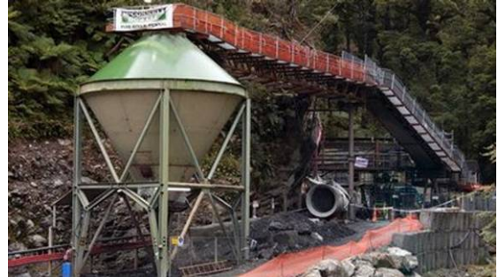
Pike workers made redundant. Photo: NZ Herald
