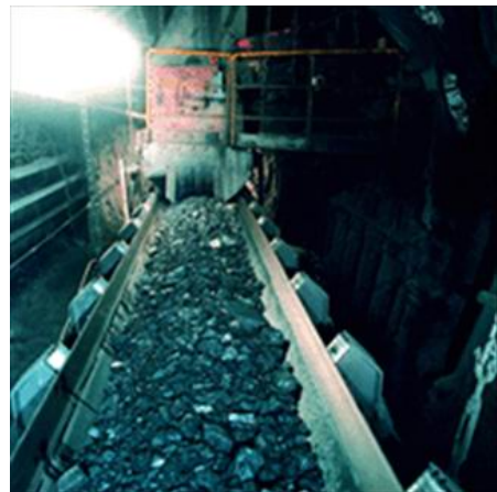
Fire resistant belt conveyor at a coal mine
