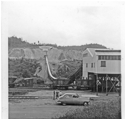
Stockrington Number 2 Colliery, No.3 Tunnel, Stockrington, NSW, [n.d.]
