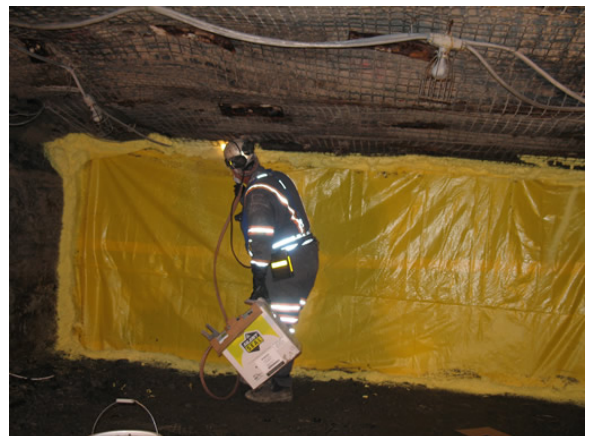
Polyurethane foam being sprayed to seal edges of brattice cloth barricade.
