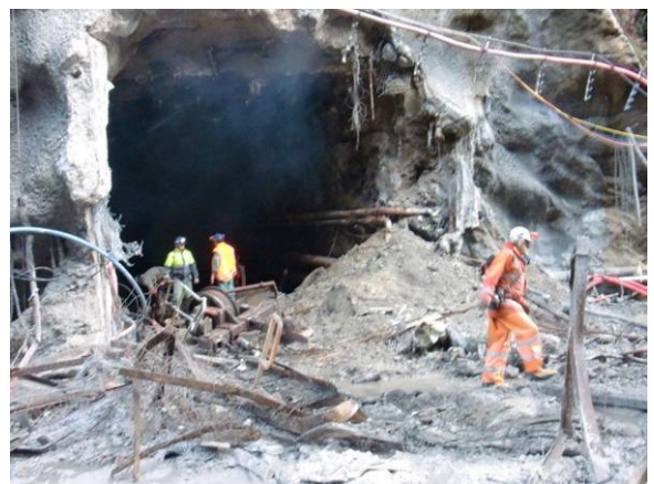
The portal seal is removed from the Pike River mine. Photo / Supplied
