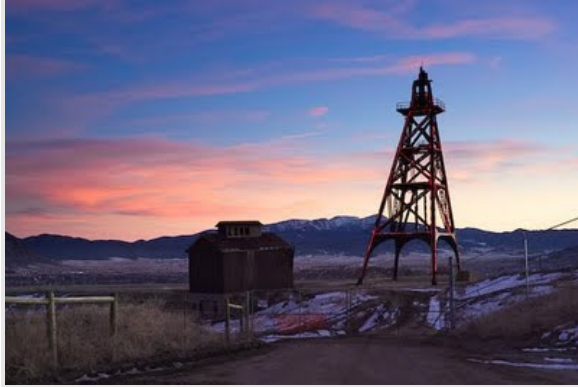
Bell Diamond Mine headframe popularly known as a "Gallus Frame" in Butte, is one of the most photographed icons of the "The Richest Hill on Earth". It now remains as a sentinel overlooking the ravages of over 100 years of mining.
