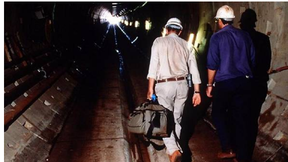
BHP workers in an underground harbour tunnel between Nelson Point and Finucane Island (file picture). Source: Supplied
