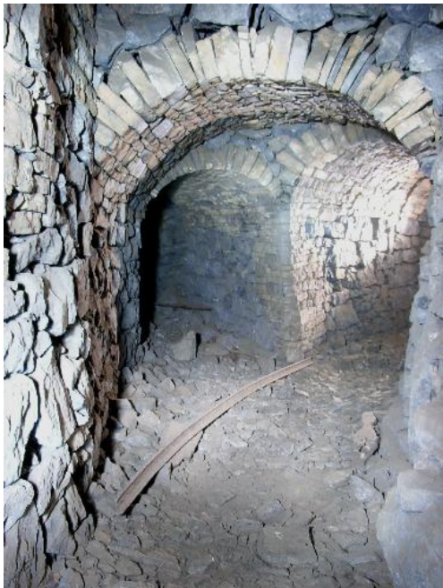
Arching underground at Smallcleugh Lead Mine, Nenthead, Cumbria, UK
