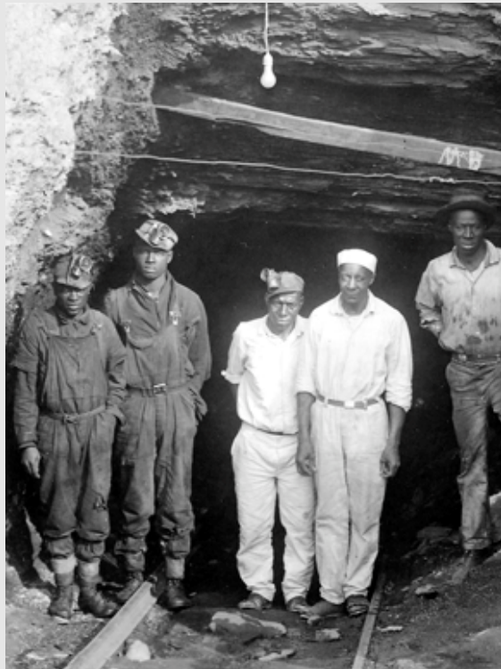
Workers at Banner Mine
