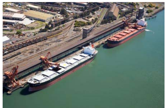
Bulk coal ships loading at Carrington Terminal, Newcastle NSW
