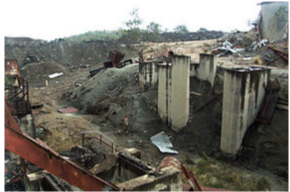
Piles of asbestos and rusting equipment at the abandoned Woodsreef mine. (NSW Ombudsman)
