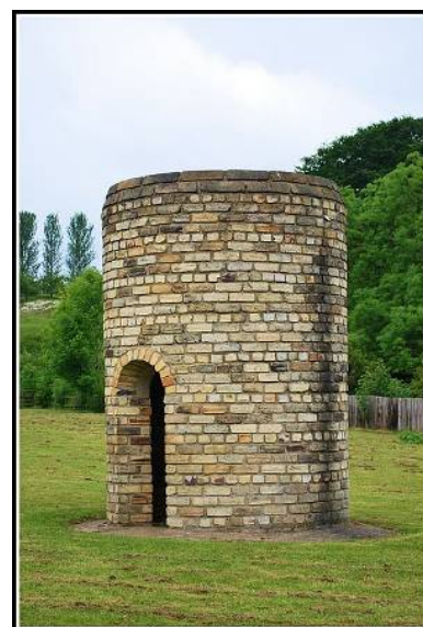
An air shaft above a coal mine
