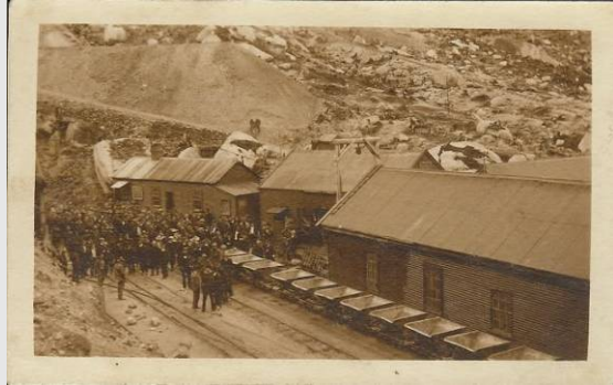
Waiting for news at the tunnel mouth, North Mount Lyell Mine, circa 1912
