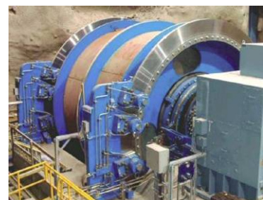
Winder, Kidd Creek Mine, Canada
