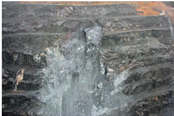
Last month's rockfall at Grange Resources' Savage River iron ore mine in Tasmania is expected to cost the company $50 million. (Grange Resources)
