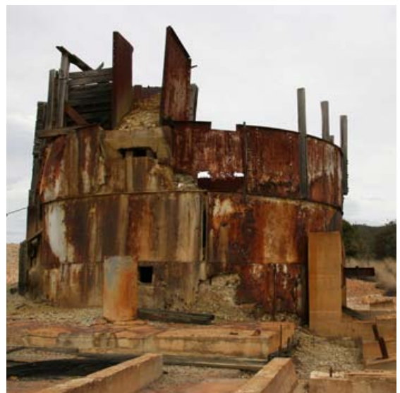
Remnants of the old days: water-jacket smelter at lead and silver mine from 1885 at Captain's Flat, east of Canberra, NSW
