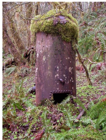
Remnants of a donkey boiler
