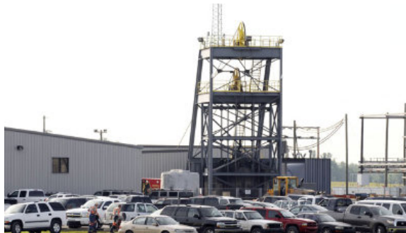
An entrance to the Dotiki mine in Hopkins County, Ky., is seen Thursday, April 29, 2010. Two employees at the Dotiki mine in Hopkins County, KY. are missing and rescuers were unable to contact them after a roof collapsed Thursday, April 29, 2010, officials said. Rescue operations are underway. (Photo AP)
