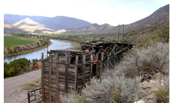
Old coal mine tipple, circa 1900s New Castle, Colorado, USA
