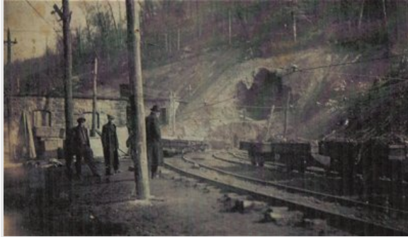
Layland mine portal after the explosion
