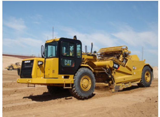
Topsoil removal for treatment
