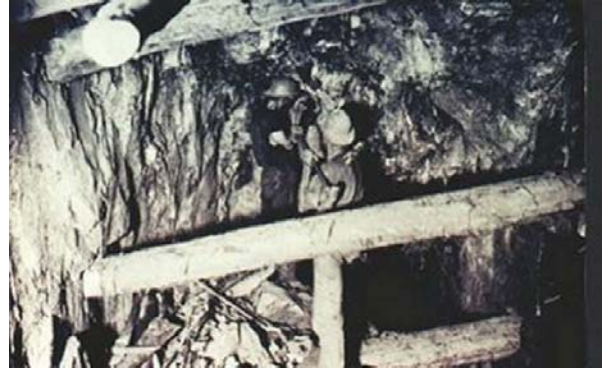
Stulls supporting a stope in a lead mine
