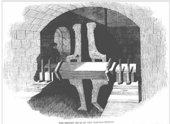
Close-up of the fractured beam
