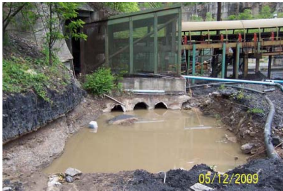
An MSHA photo shows culverts at the mine portal.
