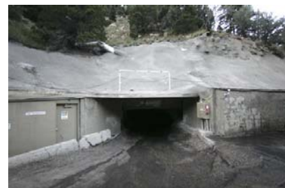
Crandall Canyon Mine adit
