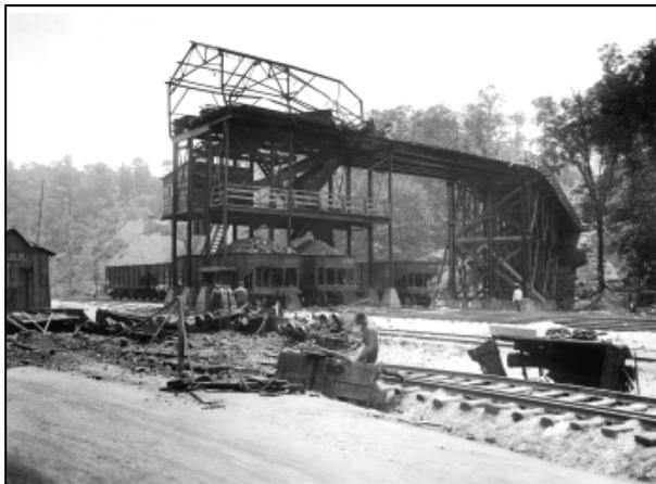
Curve in the tippel track, where the trip jumped, and the location of the wrecked trip in foreground
