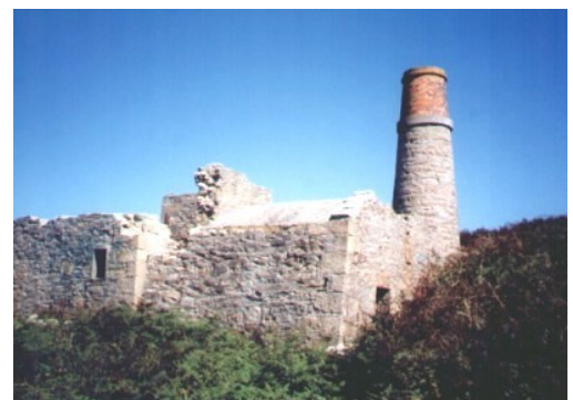
View of west and south sides of Merton furnace, Boscawell United Mine, (tin & copper) Cornwall, UK
