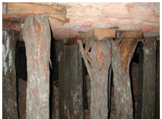
Timber props under pressure Coocoran opal fields, Lightning Ridge, NSW, circa 2001
