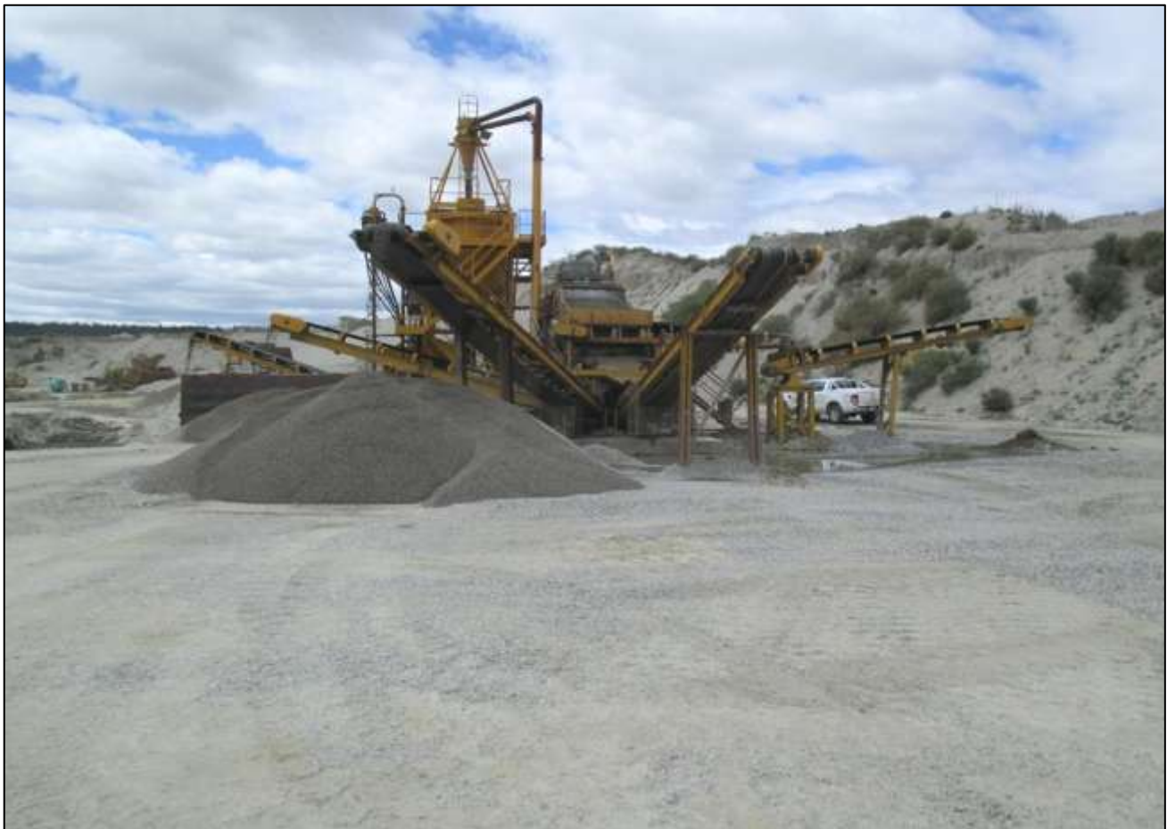
Complete Plant showing the five output conveyors.
