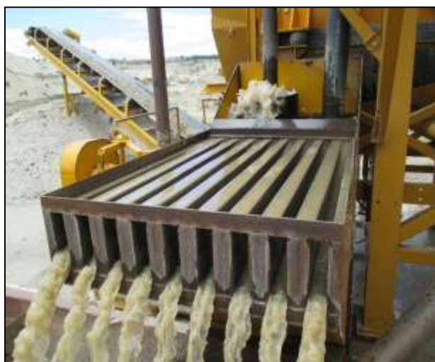
Fine Sand tank, pump and overflow weir area to retain minus 300 micron sand
