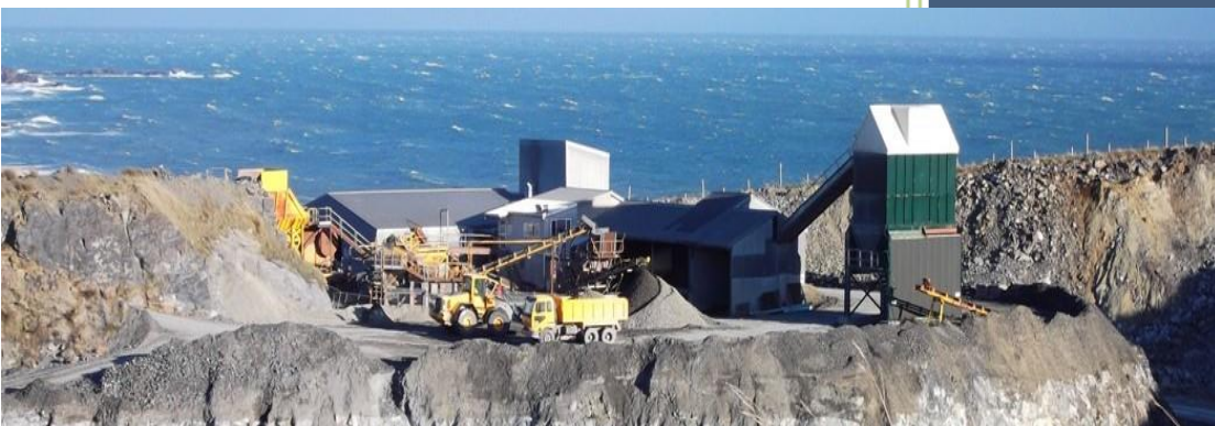
Greenhills Quarry, Bluff
