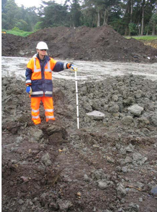
Figure 14: Ensuring mildly contaminated material is excavated to the correct depth.
