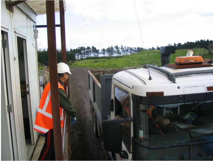
Figure 8: The fill inspector inspecting a truck load before it tips off.
