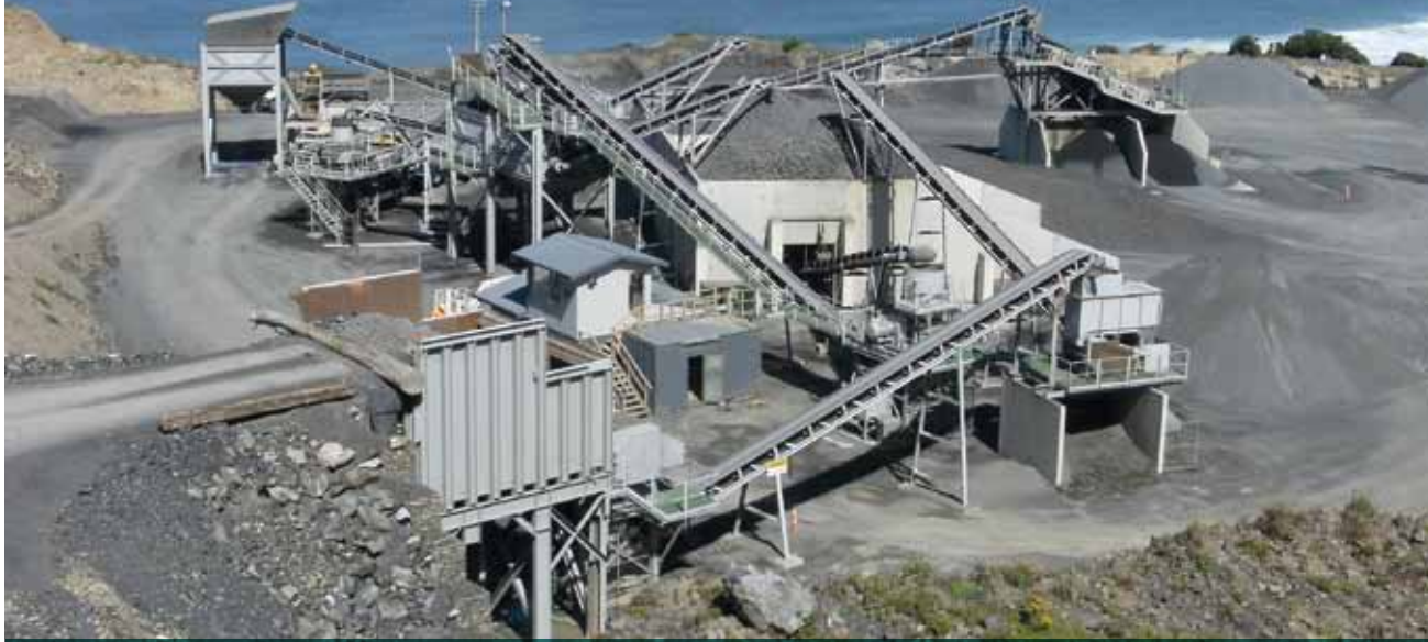
The upgraded Blackhead Quarry site – quarrying operations are carried out in a manner as natural as practicable to fit into the surrounding environment
