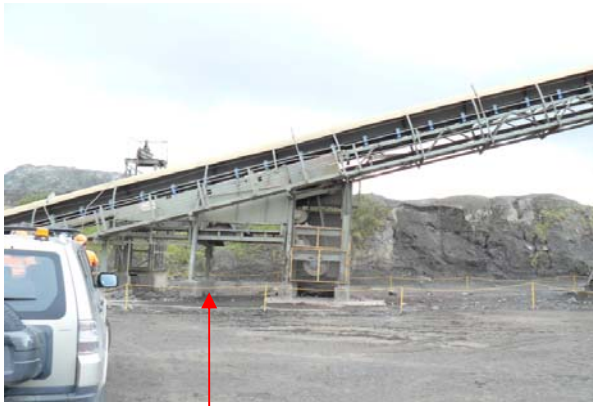
The injured worker was standing in this area when struck by the rock.
