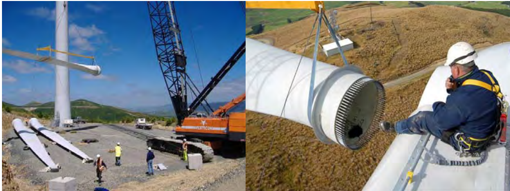
Installing the blades
