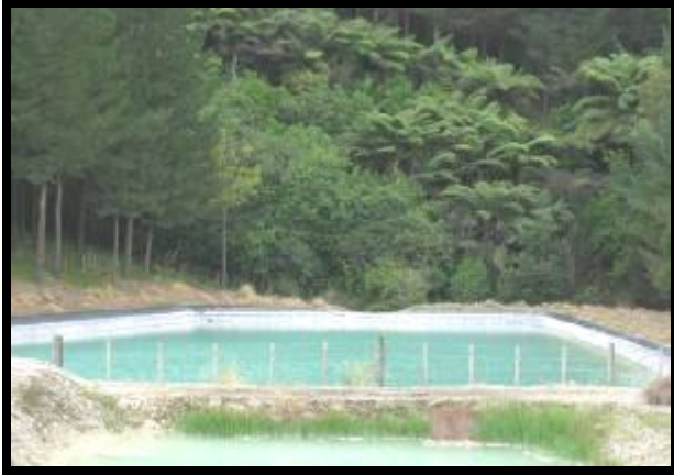
Fig. 2 Water storage / harvesting pond
